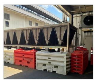
The old and new chillers were observed along with the chiller pumps. The old pumps will remain once the new chillers are put in place. *Chillers are new and in good condition. The chiller area is clean and well maintained.*
